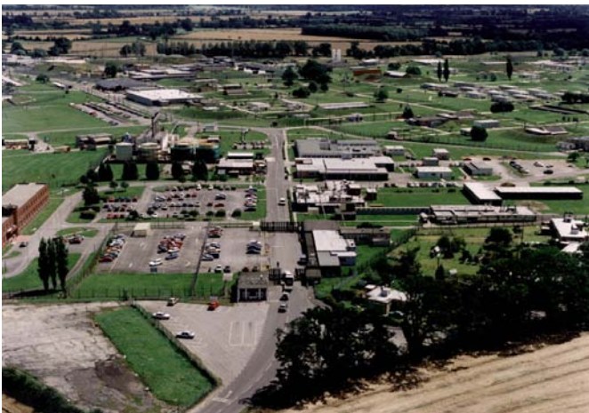
AWE Burghfield, main entrance
